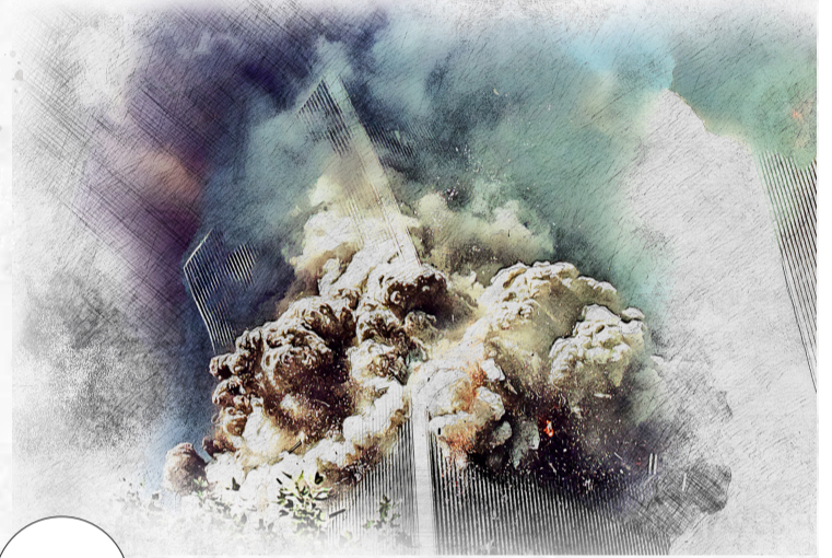
9:59 am The World Trade Center's heavily damaged South Tower collapses.
